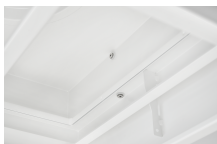
Pressure measurement point, detail
