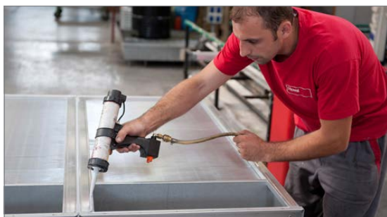
Fgi. 3: Apply sealing compound
