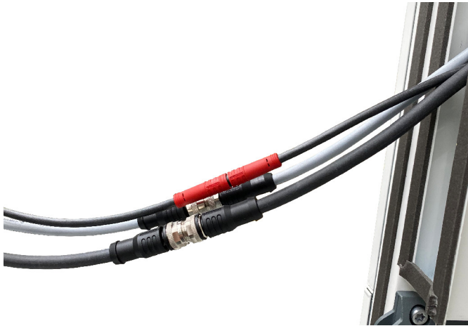
Fig. 41: Connection of the cables
