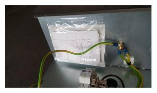
Connect the unit according to the wiring diagram.
