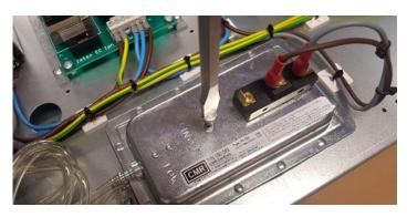
Slowly turn the screw back CCW until the heater Relay or Contactor energizes again.
